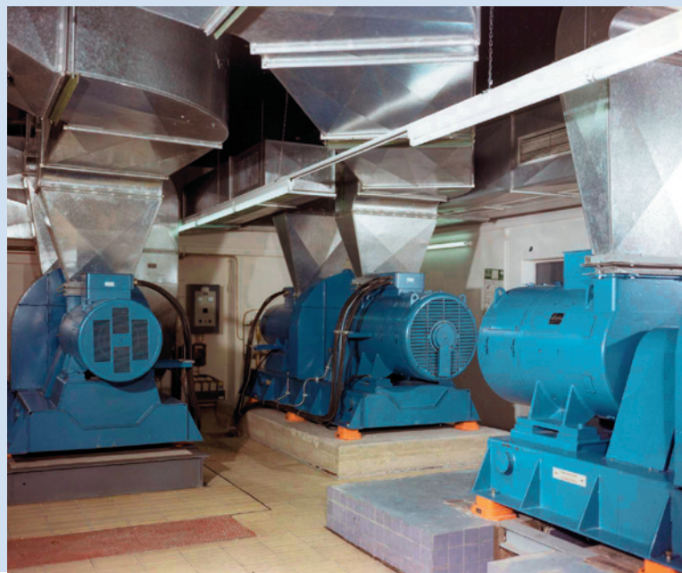
Air Conditioning System with Spring Units
