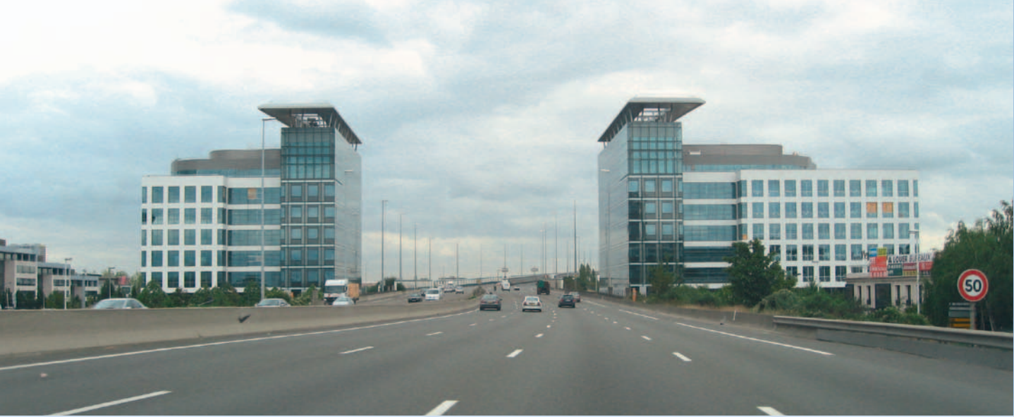
2 spring supported buildings close to an elevated city highway – Paris, France
