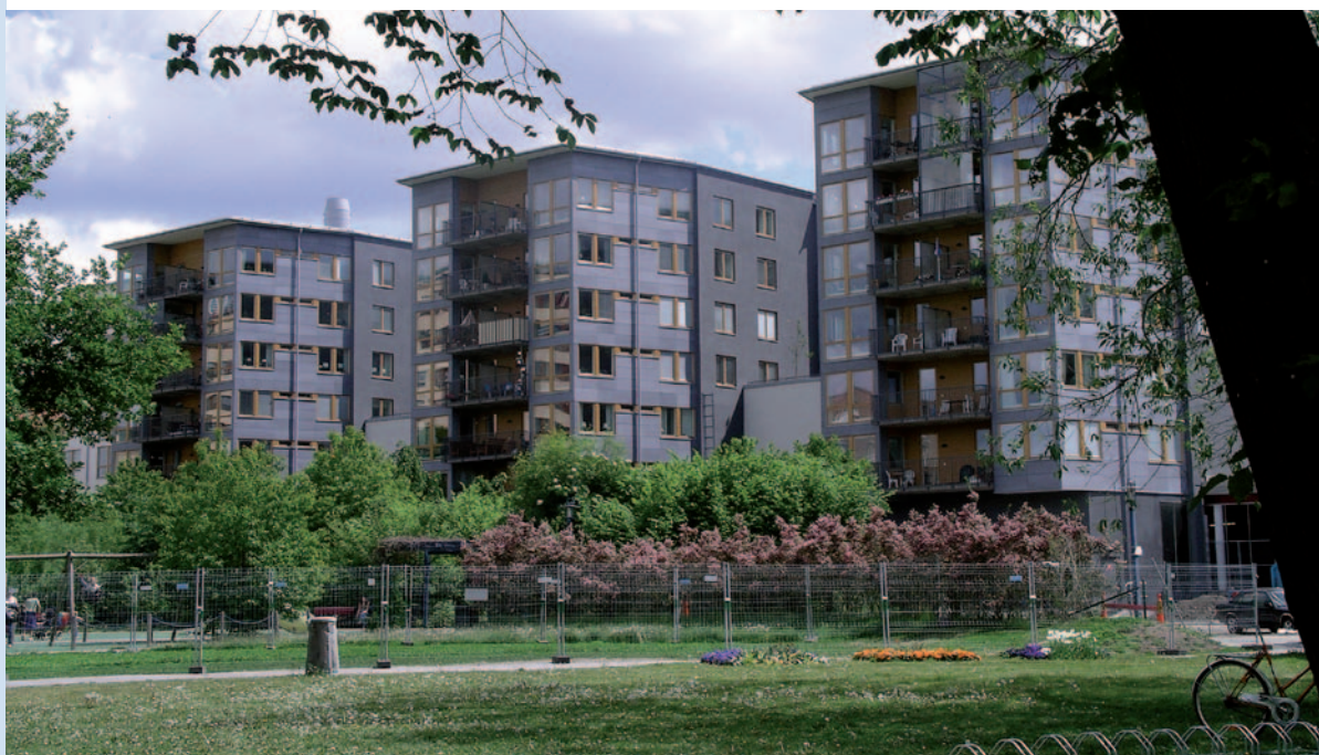
Residential buildings, partially spring supported on top of a railway station – Stockholm, Sweden
