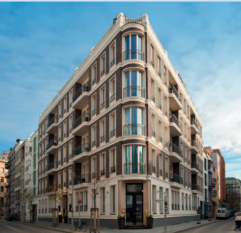
Spring supported residential house – Berlin, Germany
