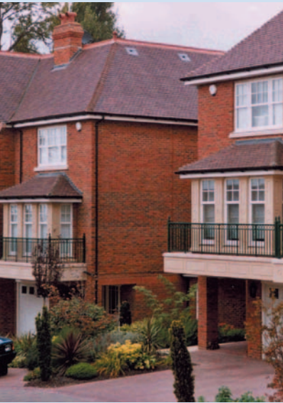
Residential houses with 3.5 Hz isolation system – London, GB
