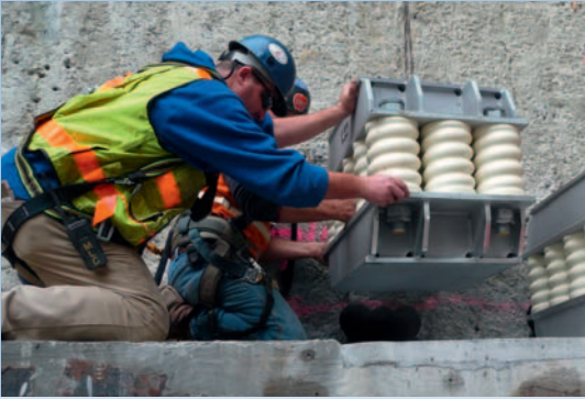
Positioning of prestressed spring elements – Boston, USA
