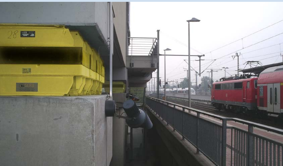
Spring supported cinema building close to a railway station – Siegburg, Germany
