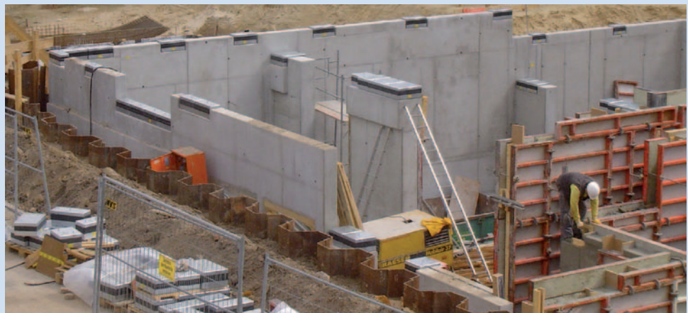
Vibration isolation of a townhouse above metro line – Berlin, Germany
