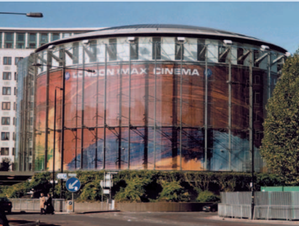
IMAX Cinema with 3.5 Hz isolation system – London, GB
